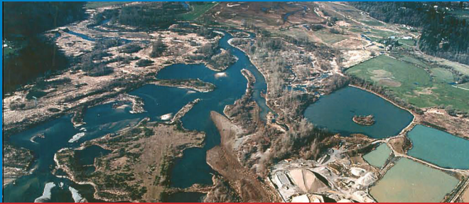
Lower East Fork Lewis River Lasting Damage and Breaching from Mining
